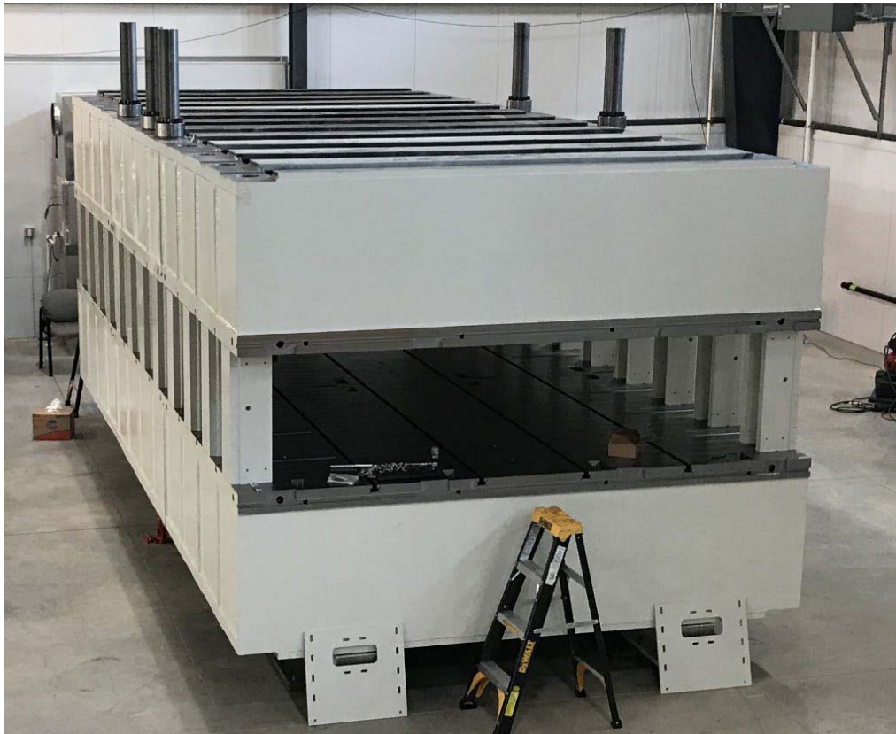
Figure 44. Lower and upper restraint elements in place and columns installed
